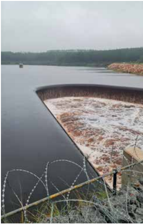
The Garden Route Dam overflowed for the first time since its spillway had been raised in 2019. The award-winning bill-shaped design increased the dam’s overall capacity by 25% by raising the spillway by only 2.5m. Photo: Wessel van Heerden
