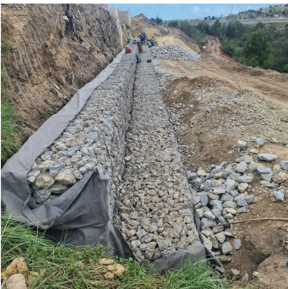
At the Schaapkop Pump Station, the slope on the river bank is being stabilised and rehabilitated.
