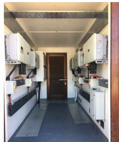
All of the inverters which will convert DC power from the panels into AC electricity have been installed in a closed-compartment room.
