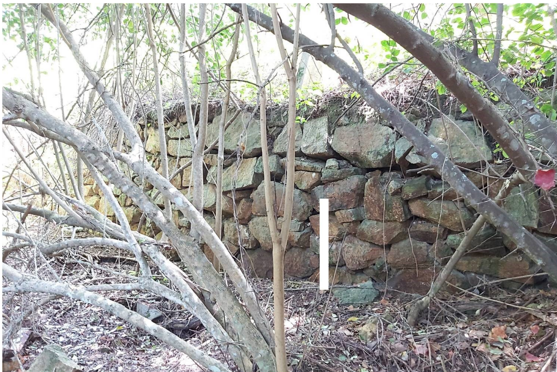
Figure 18. Example of best preserved part of stone walling. Scale bar is 100cm (1m) long. (A4 version on pg 56)
