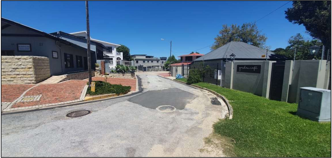
Figure 3.5 Sight distance looking right
