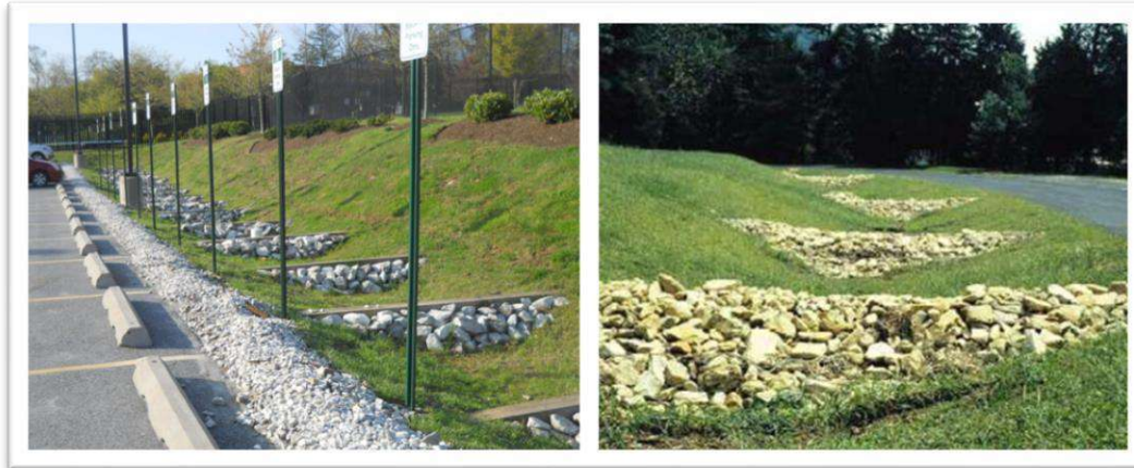
Figure 3-3 - Examples of Stepped Energy Dissipaters
