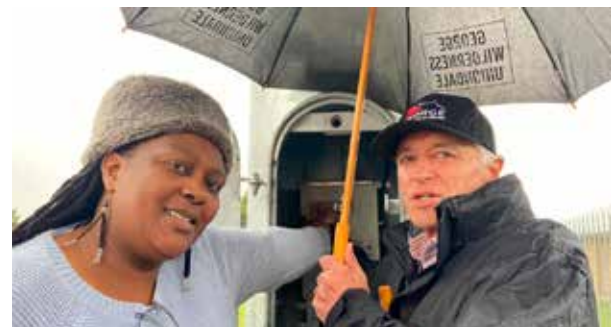
At the switching on of a High Mast light in Nel Street, Borchersds are Mayor Leon van Wyk and Cllr Nosicelo Mbete, Portfolio Councillor for Electrotechnical Services and Fleet Management.
