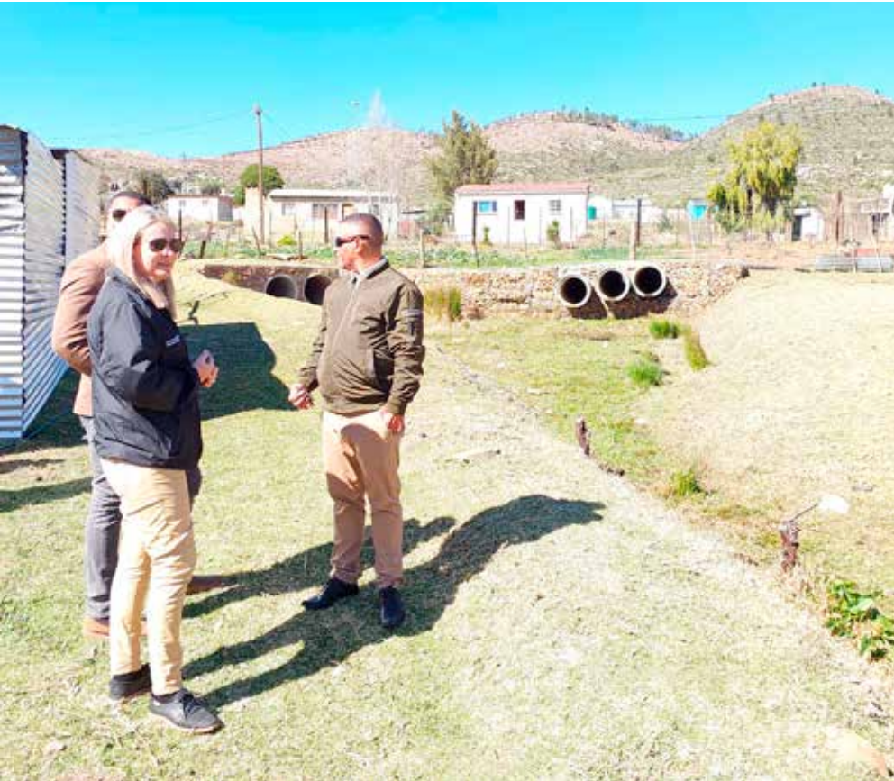
In the photo is the Executive Mayor, accompanied by Cllr Justin Fry (Ward 25, Haarlem) and Cllr Browen Johnson, MMC Civil Engineering Services, visiting a resident's house, Evelyn Thyse. Thyse has an issue with the stormwater pipes in the photo, which often cause flooding on her property. Deon de Jager, Deputy Director of Civil Engineering Services, was also part of the delegation to make recommendations.
