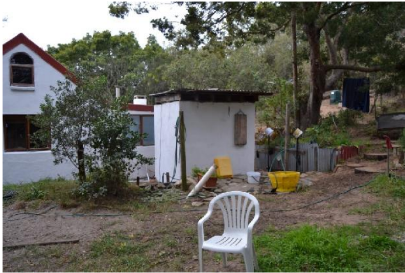
Picture 2. Existing laundry room
