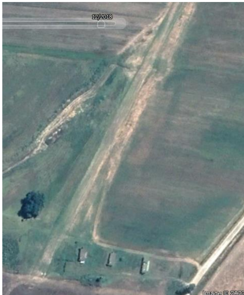
Fig. 3 : 12/2018 : N/S runway lengthened to about 450m
