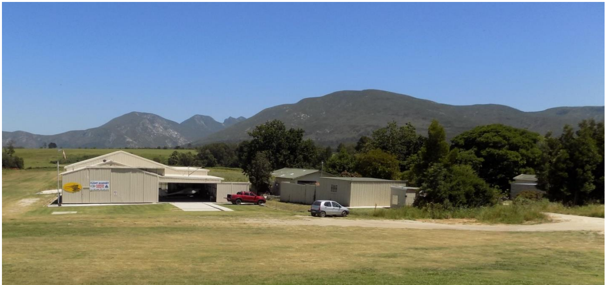
Fig. 12 : 11/2023 New hangar added north (right) of existing building.
