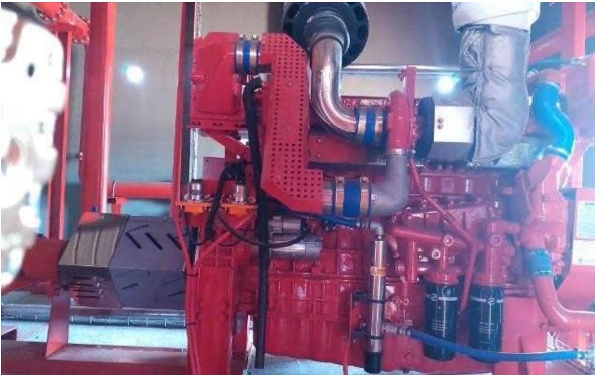
Diesel driven fire pump.
