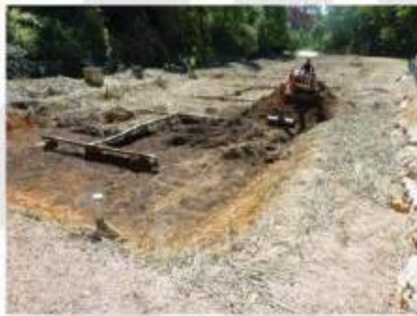
Composted sludge removed from first stage of Phragmifiltre after 14 years - Roussillon, France
