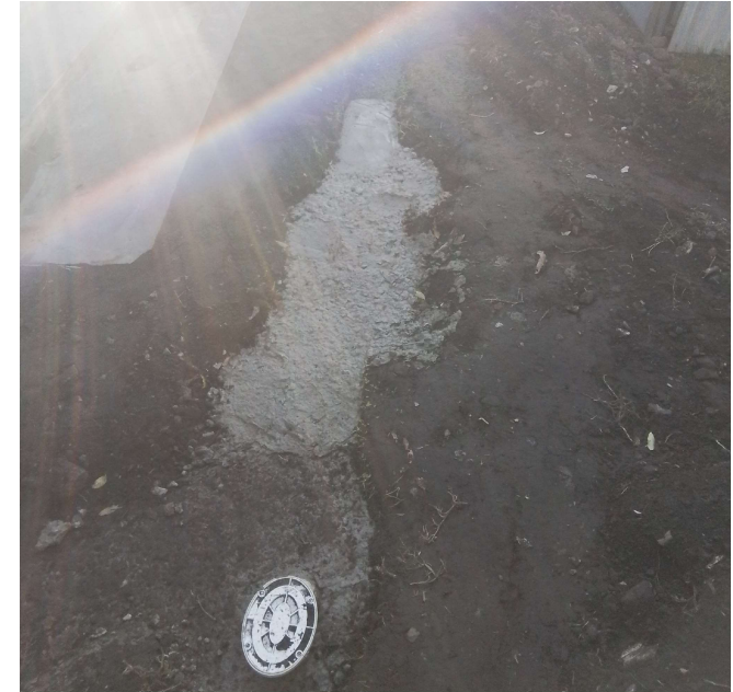
Trench and pipe covered in concrete before being inspected.
