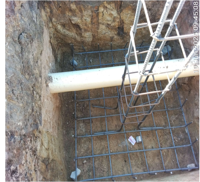
Sewer line running under and through foundations. Services in a trench.
