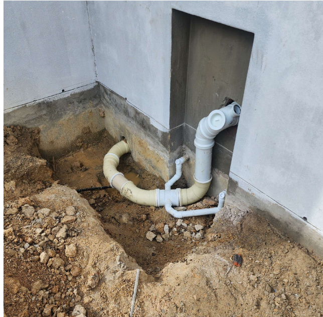
40mm waste plumbing not according to the Approved plan layout.
