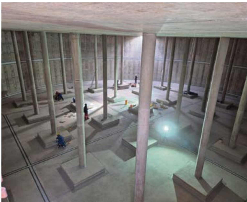
Inside Thembalethu East Reservoir.
