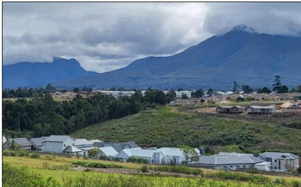
FIGURE 18: WELGEVONDEN DEVELOPMENT, WITH GROENKLOOF IN THE BACKGROUND
