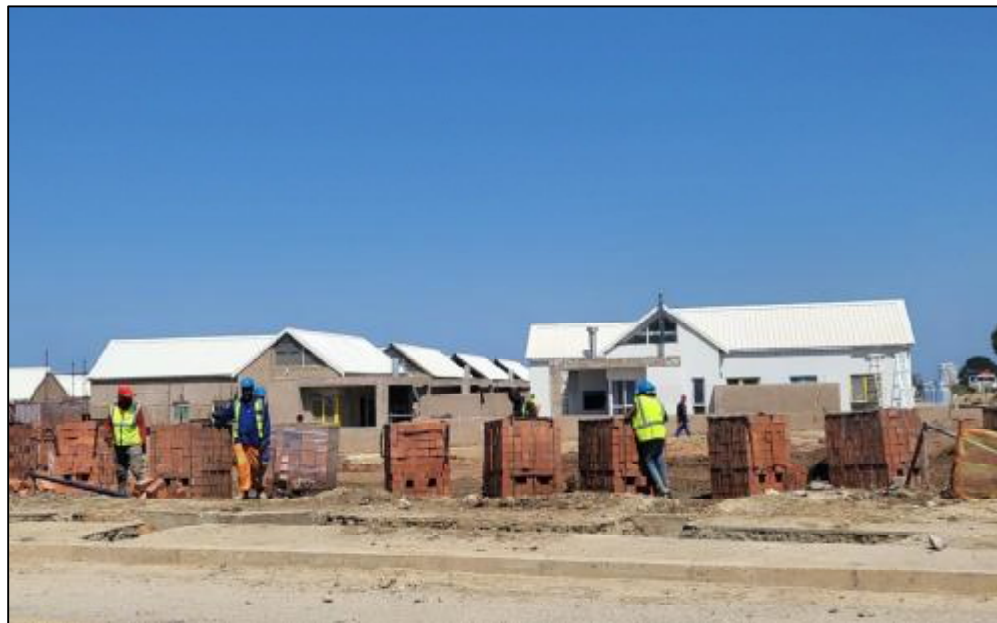
FIGURE 16: HOUSES UNDER CONSTRUCTION IN SPRINGFIELD ESTATE
