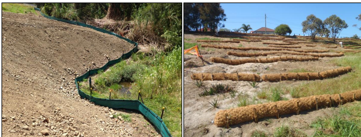
Figure 16: Examples of silt fences (left) and coir logs (right) used to trap sediment mobilised from steep slopes.
