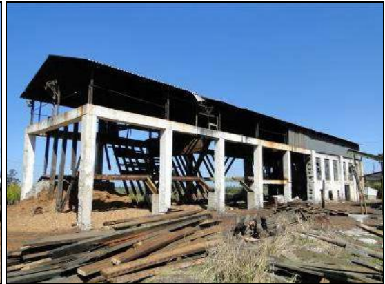
Image 5: North-facing elevation, boiler, cyclone no longer in place. V-shaped hopper partly removed
