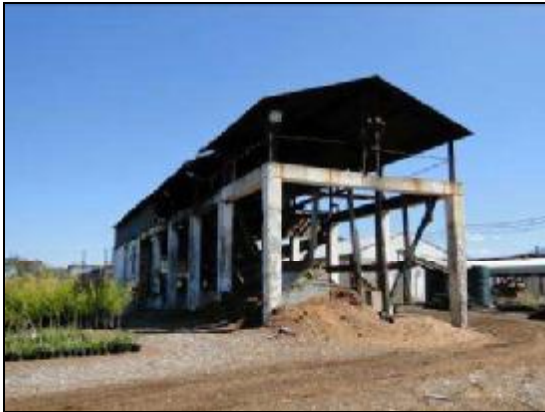
Image 4: East-facing view of former Boiler room
