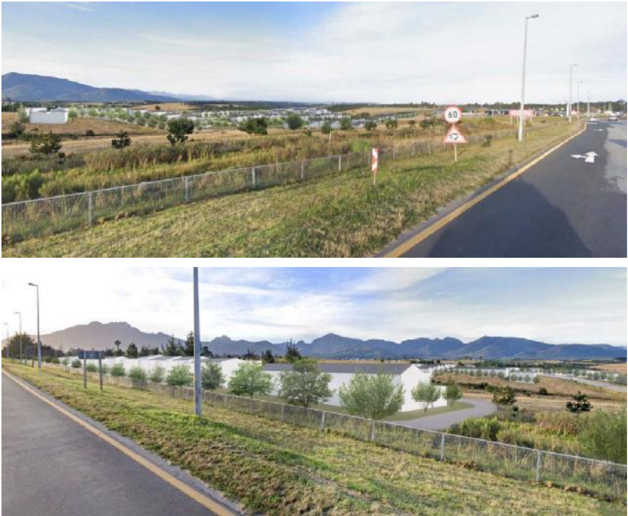
Figure 7: The key views that will need to be taken into account are from the N2 Highway section (NuVorm, 2025)
