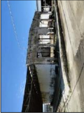
Photo 13: Concrete block building fitted with steel window frames.
