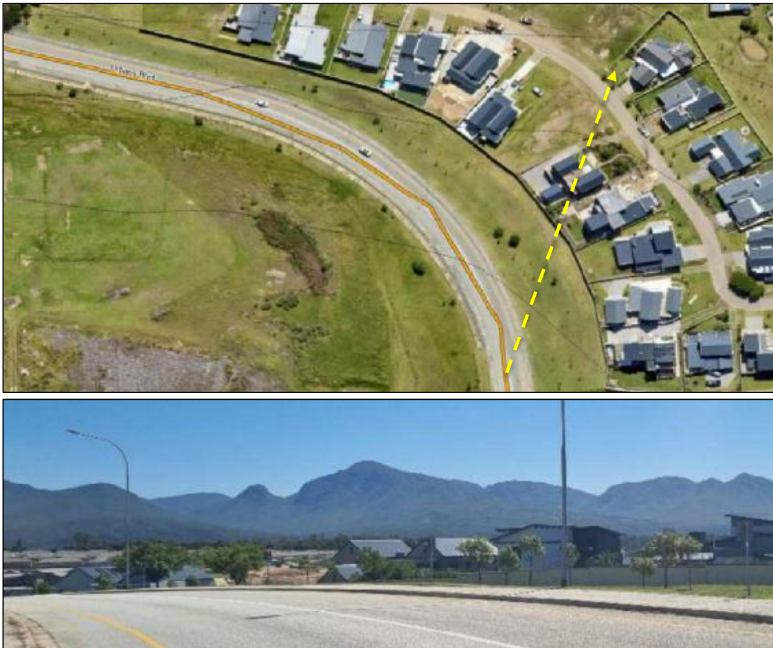
Figure 18. Welgelegen Estate to the northeast of the Urbans Boulevard with suitable development precedent from views over the structures that are well set back from the road.
