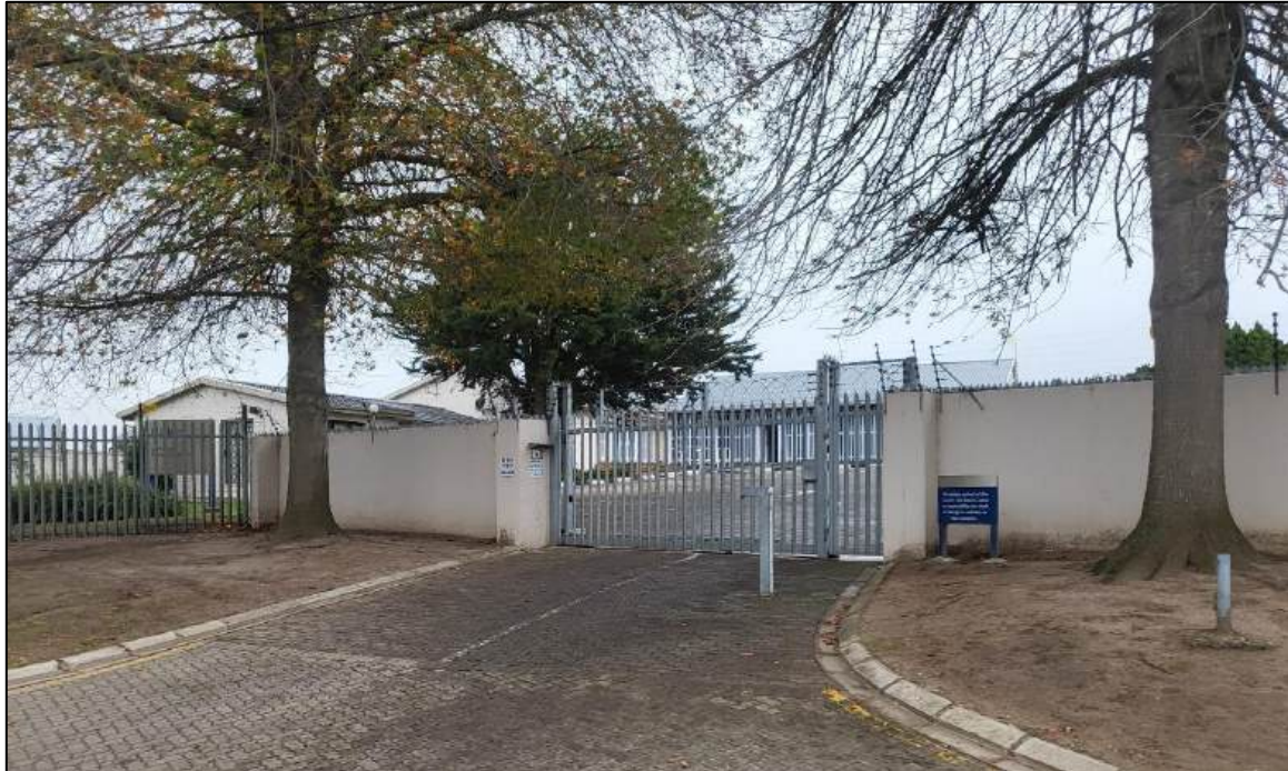
FIGURE 10: ESKOM OFFICES ON PORTION 43 OF FARM NO 212
