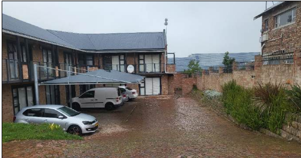
FIGURE 6: EXISTING BOARDING HOUSE ON THE APPLICATION AREA
