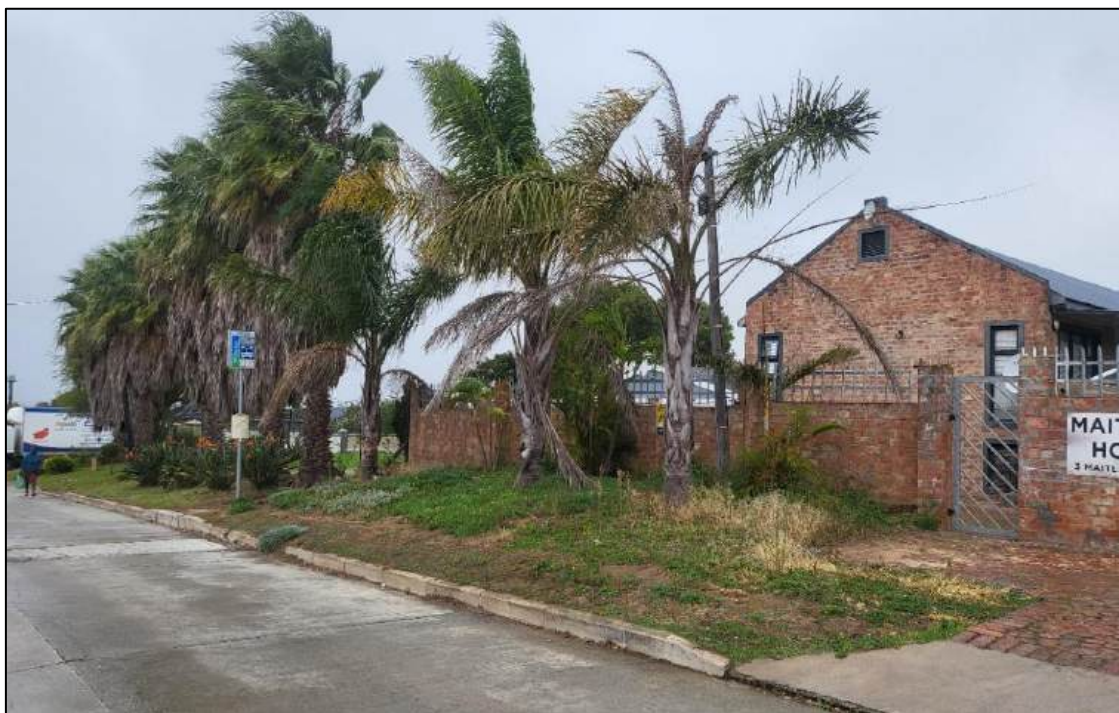
FIGURE 1: GOGEORGE BUS STOP AT THE APPLICATION AREA
