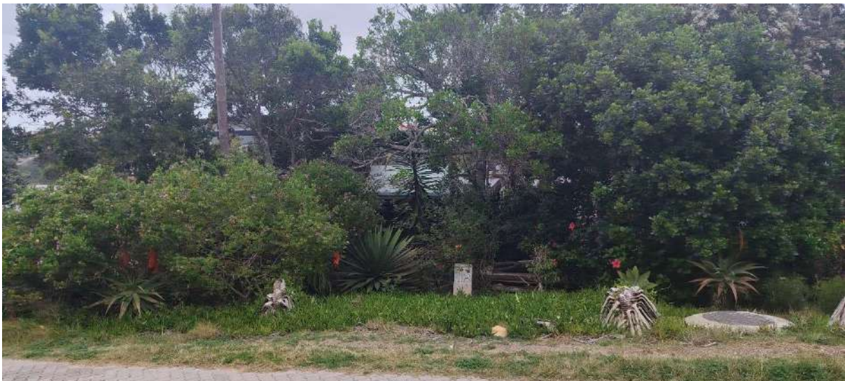
Photo 4 This photo was taken from the adjacent street directly towards the unfinished toolshed the owner was busy to erect when a notice was served on him. This building can be seen more clearly on photo 5 below. Note that as a result of the vegetation on the erf, the structure is barely visible. This building has in the meantime been demolished. The structure on the left side of the photo, is the dwelling house on the neighbouring property.
