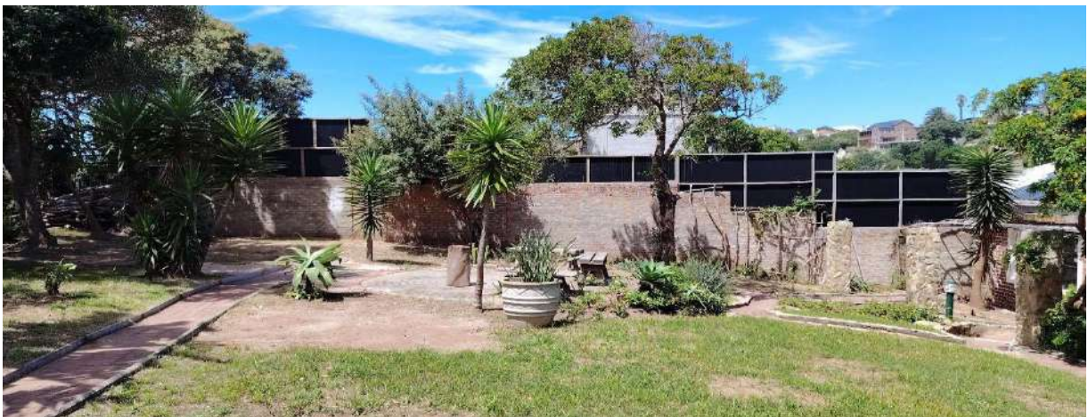
Photo 6 This photo was taken from almost the same position as photo 5 above and shows that the unlawful outbuildings as well as the timber deck that was attached to the main building, have already been demolished. The Boundary wall and screening that are mentioned in paragraph 5.3.4.1.1 below, are also clearly visible after the demolition of the outbuildings.
