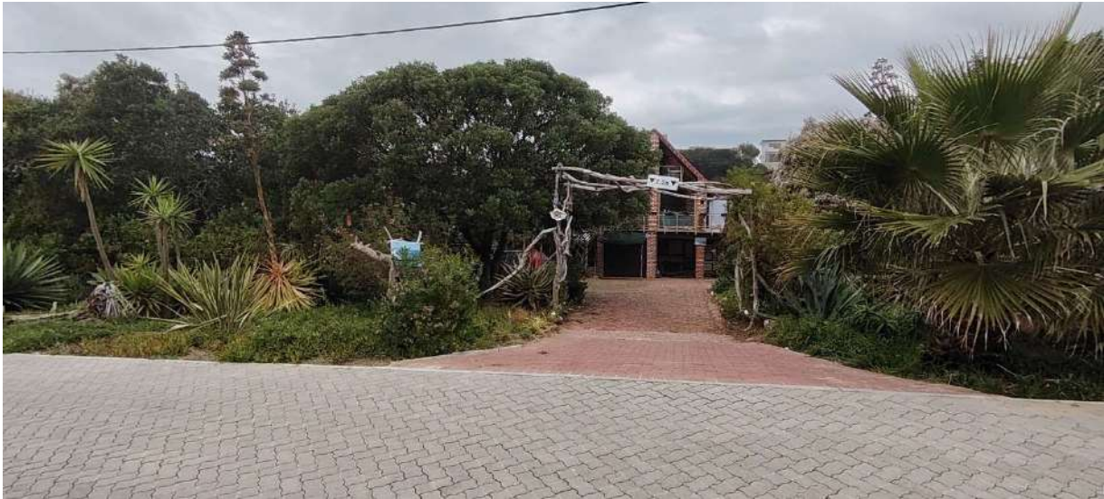
Photo 3 The existing dwelling house on Erf 754 as seen from the street outside the erf in a southerly direction. Note that much of the building is hidden from the street by the existing vegetation on the property.
