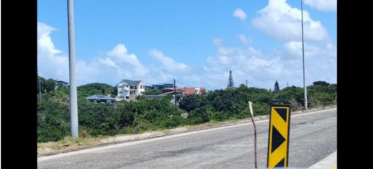
Photo 15 This photo was taken from the N2 travelling in a westerly direction. The photo was taken in a south-westerly direction and shows how the dwelling on Erf 754 (the red roofed building in the center of the photo), is in fact dwarfed by buildings behind it that really break the skyline and is very visible from the N2. The dwelling on Erf 754 is barely visible from this direction.
