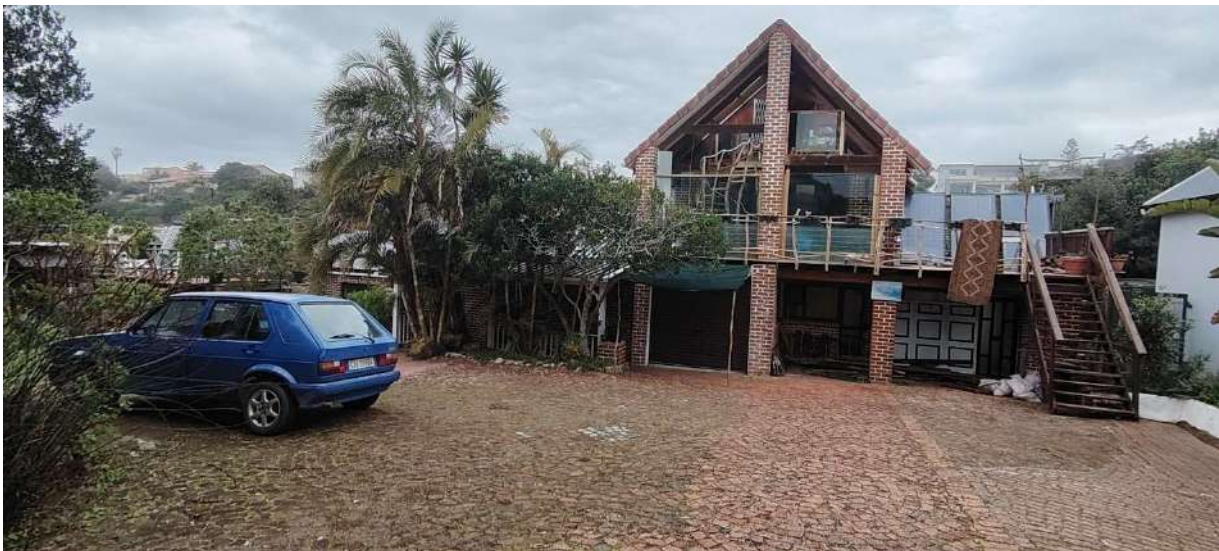
Photo 2 The existing dwelling house on Erf 754 as seen from inside the erf in a southerly direction. On the right side of the photo, the south-eastern corner of the dwelling on Erf 753 is visible. Also see photo 6 below.
