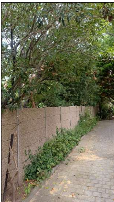
Figure 15: Boundary wall to the southern neighbour
