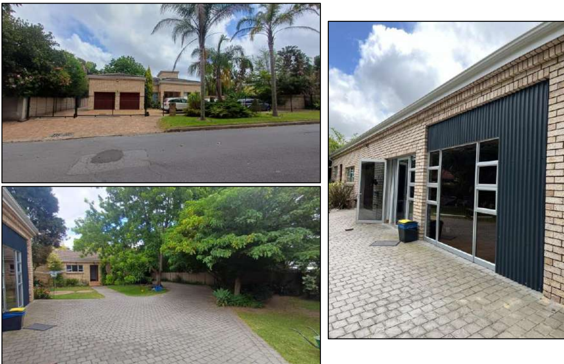
Figure 3: Existing structures and character of the subject property
