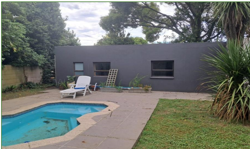
Figure 4: Existing encroaching structure
