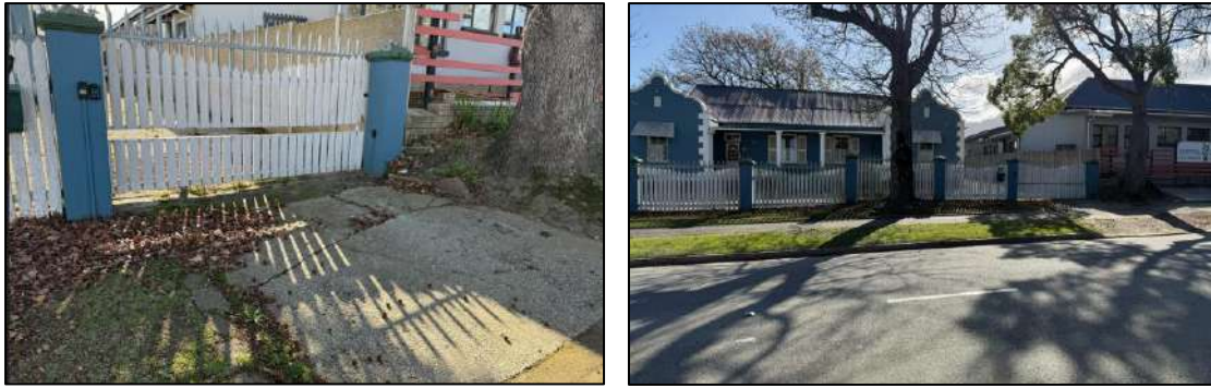
FIGURE 6: EXISTING ACCESS FROM MONTAGU STREET
