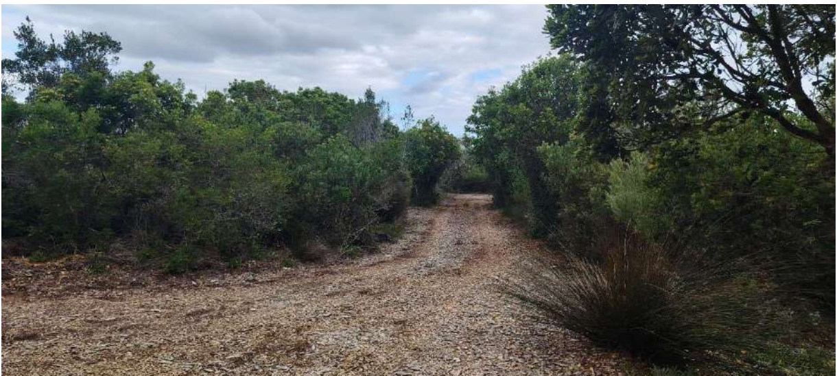
Photo 4 A section of the existing access road on the property. The covering on the road surface is wood chips that is very eco- friendly in this type of situation. Also note the indigenous vegetation that the owners have left untouched as far as possible and limited the removal thereof to a minimum.
