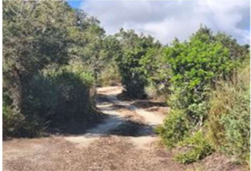
Figure 3 Existing Access Road
