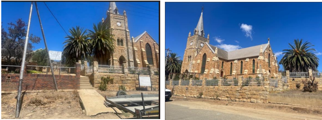
Photo 3: View of the Church Hall and offices, and Church building from Hood Street
