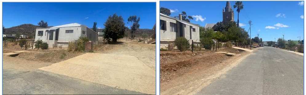
Photo 15: Stormwater system in Hood Street
