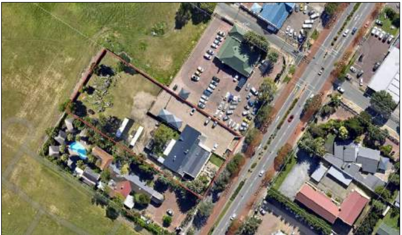
Figure 2: Enlarged aerial photograph
