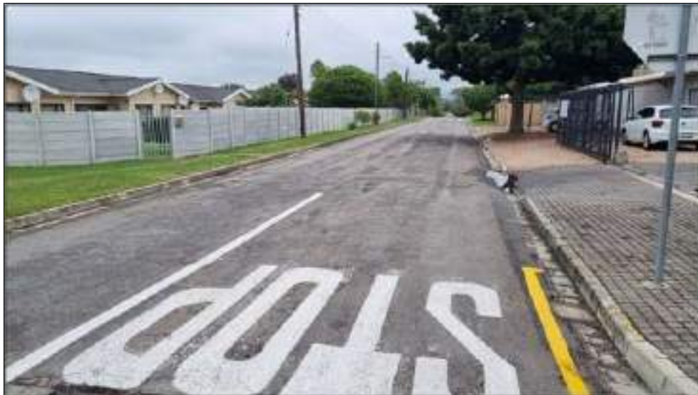
Photo 3A: Looking north-west along Belvedere Rd from York St
