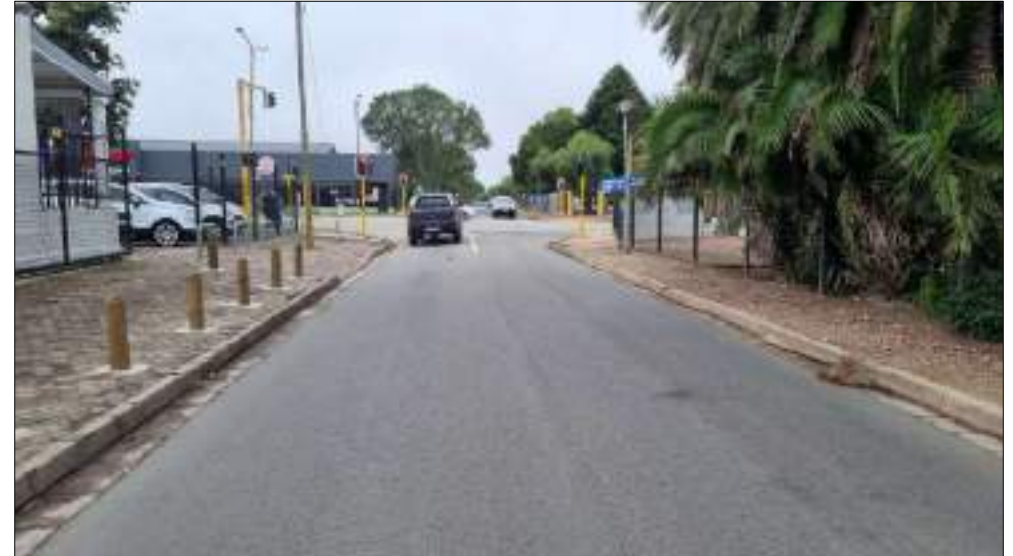
Photo 2B: Looking south-east along Fichat St towards the York St intersection
