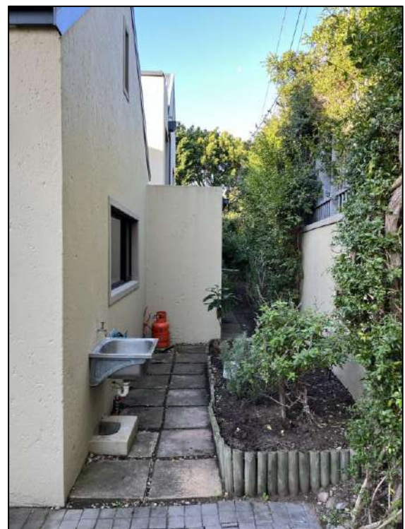
Figure 4: As-built existing addition
