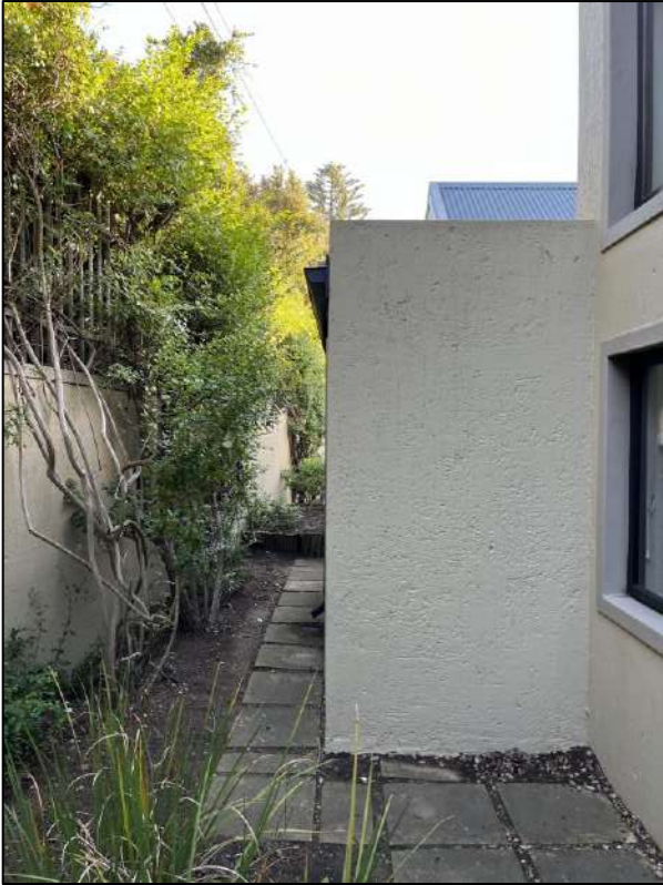
Figure 6: Visual along the rear side
