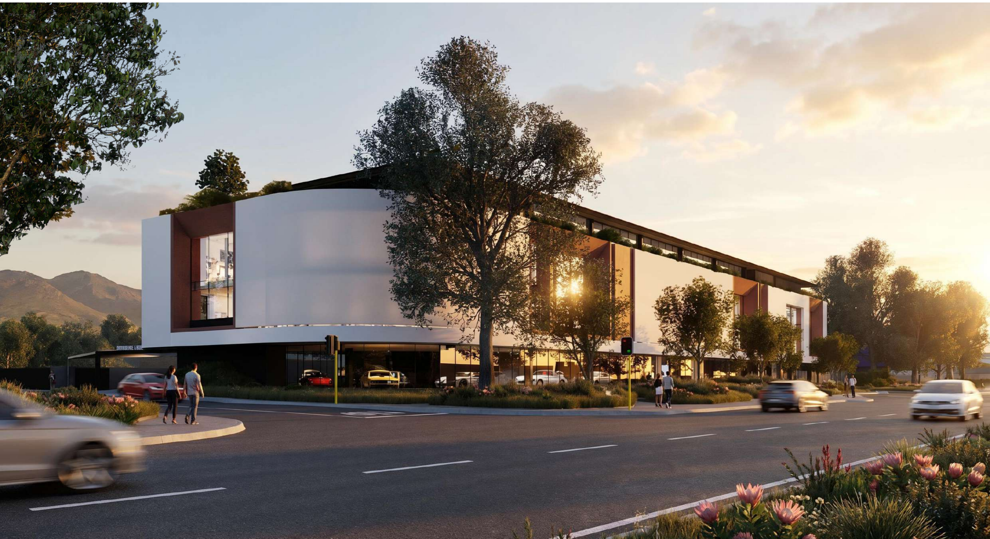
CORNER VIEW OF KNYSNA RD AND 3 rd STREET
