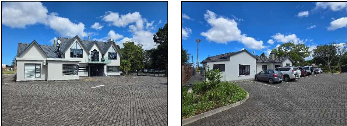
FIGURE 5: EXISTING BUILDINGS ON THE APPLICATION AREA
