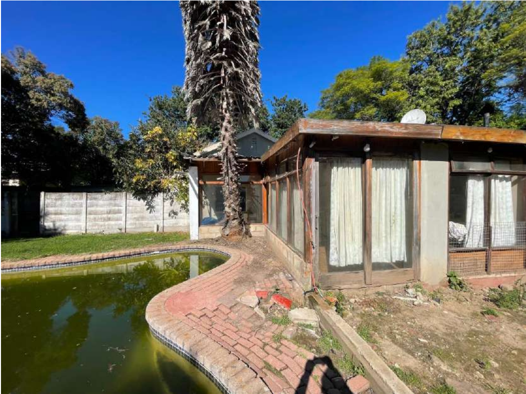
Facia boards and window and door frames rotted through. Gutters in poor state. Door and window frames have not kept the house sealed for many years. Water damage internally evident.
