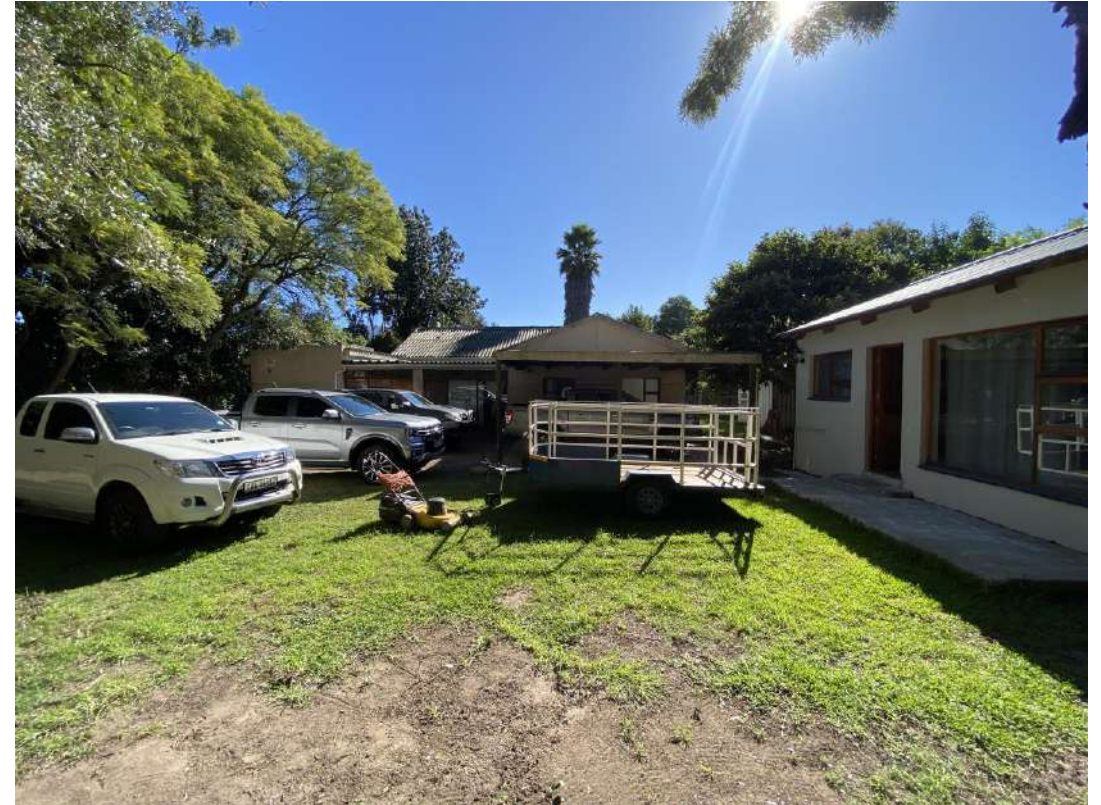
Roof in back background rusted through and has lifting seams. Leaking over time has damaged the structure beneath.
