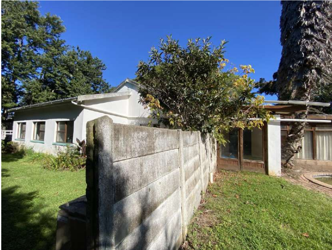
East view of existing house - window and door frames rotted through. Gutters in poor state. Wall finishes poorly maintained, showing evidence of severe damp damage as well as vibacrete wall starting to collapse.
