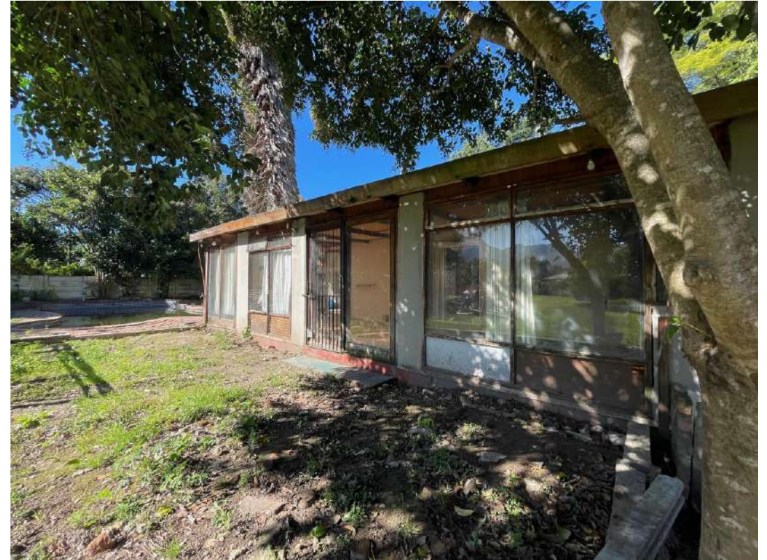
Facia boards and window and door frames rotted through. Gutters in poor state. Wall finishes poorly maintained, showing evidence of severe damp damage.
