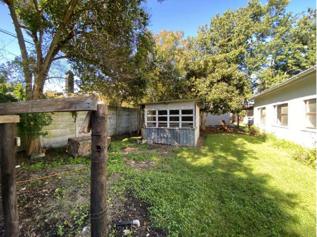
Dilapidated shed in poor state with no heritage significance
