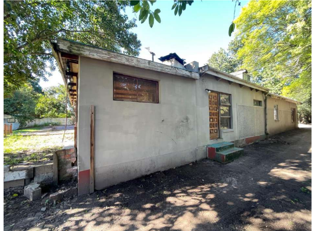
ERF 592 – Existing House older than 60 years
