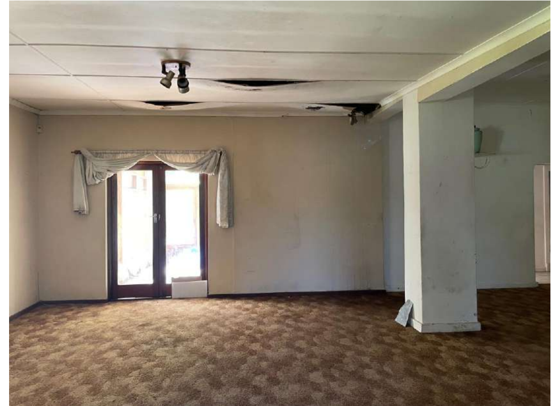
The structure is very damp inside. Ceilings are also collapsing due to water damage. No maintenance has been done for years.
