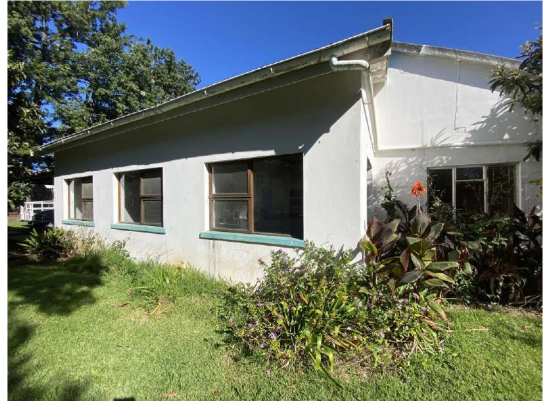
East view of existing house - window and door frames rotted through. Gutters in poor state. Wall finishes poorly maintained, showing evidence of severe damp damage as well as vibacrete wall starting to collapse.
