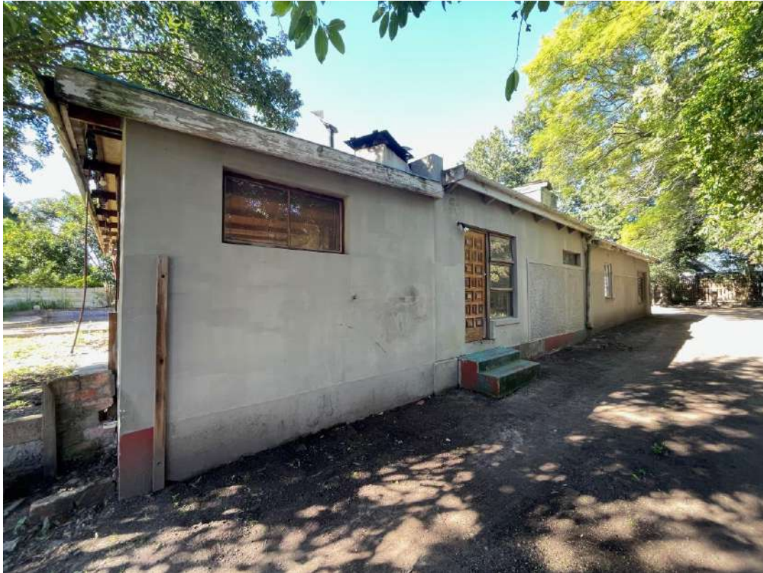
Facia boards and window and door frames rotted through. Gutters in poor state. Wall finishes poorly maintained, showing evidence of severe damp damage.
