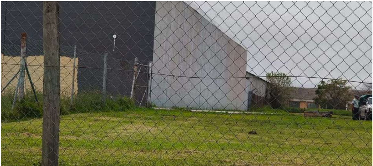
Photo 7 The photo shows another building in the industrial area that was erected on the boundary of the erf.
