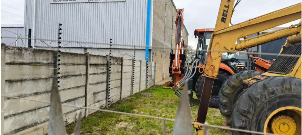
Photo 8 The photo shows another building in the industrial area that was erected on the boundary of the erf.
