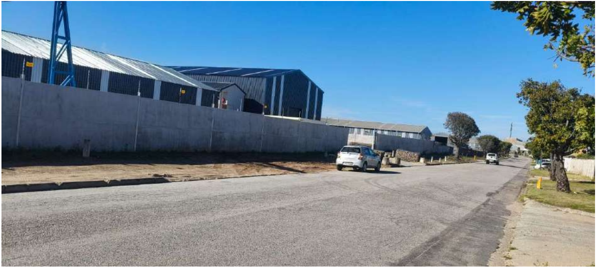
Photo 3 The photo shows the wall along Ring Road boundary on the western side of the erf. Existing buildings on the erf is also visible.
