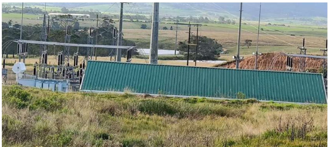
Photo 17 This photo was taken from the N2 close to the position of where photo 16 was taken in the direction of the dam on Farm 62/226. Note that the tourist units next to the dam cannot be seen from this direction although the dam is visible. The photo also shows the contrast of some structures next to the N2 compared to the rest of the agricultural landscape as seen on photo 16.
