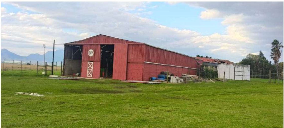
Photo 4 The farm-shed in the north-eastern corner of the farm that encroaches the property boundaries of Ptns 31 & 63 of Diepe Kloof.
