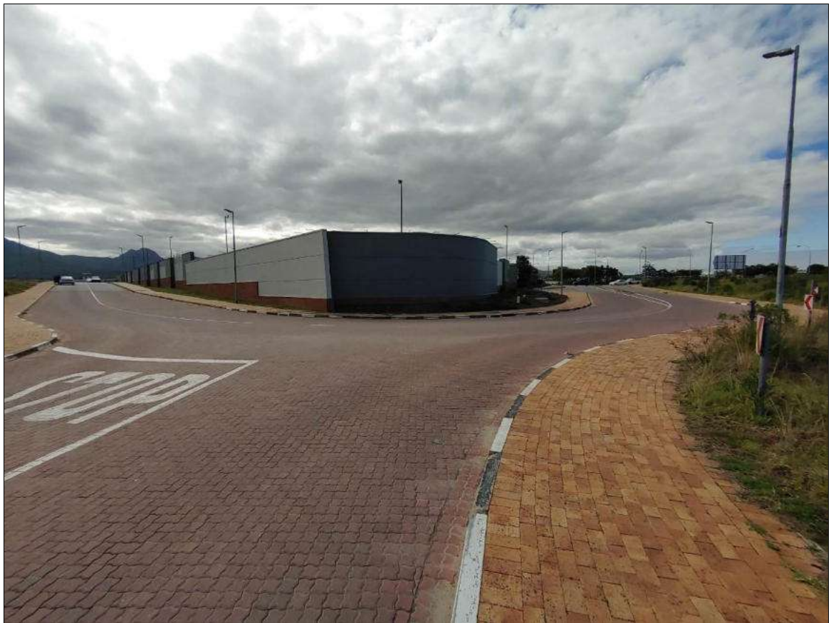
Figure 13: Existing intersection of Platinum Drive and Park Road, future traffic circle
