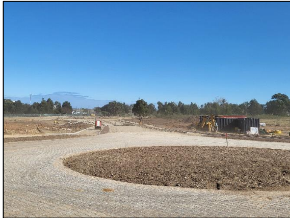
FIGURE 24: NEW DEVELOPMENT UNDER CONSTRUCTION ON PORTIONS 60 & 139
