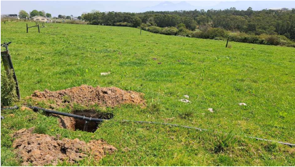
Figure 4. Typical site conditions looking west towards airport and showing excavated soil.
