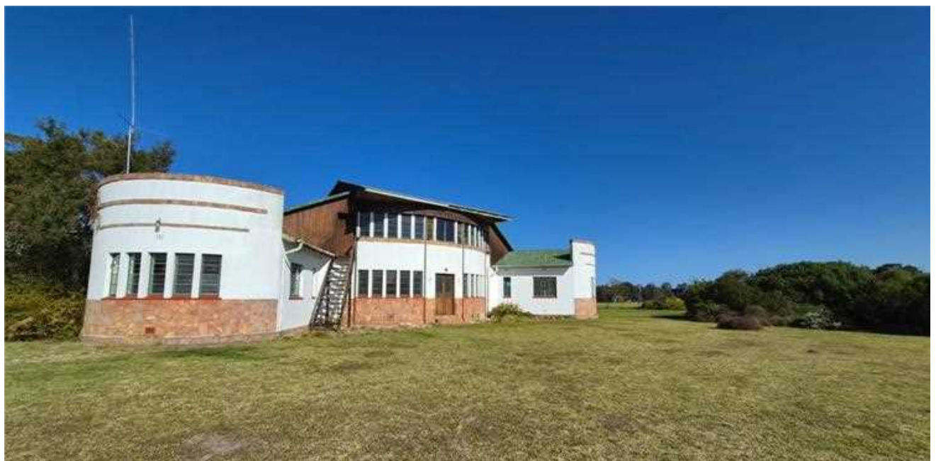
Photo 1: Building A, the original farmhouse, proposed to become a guesthouse.
