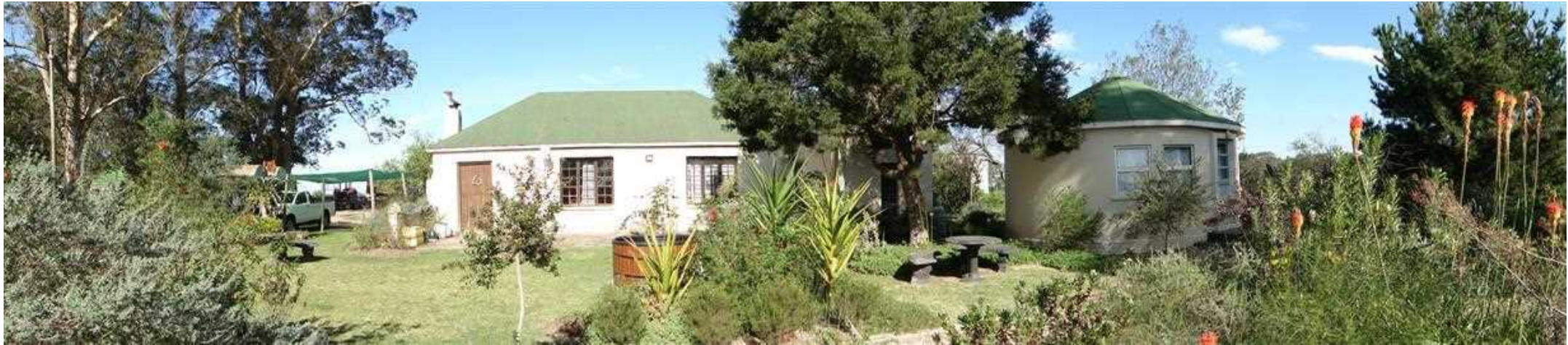
Photo 14: Main, north-facing facades of much altered former historic school building, repurposed as an additional dwelling with rondawel to the right.
