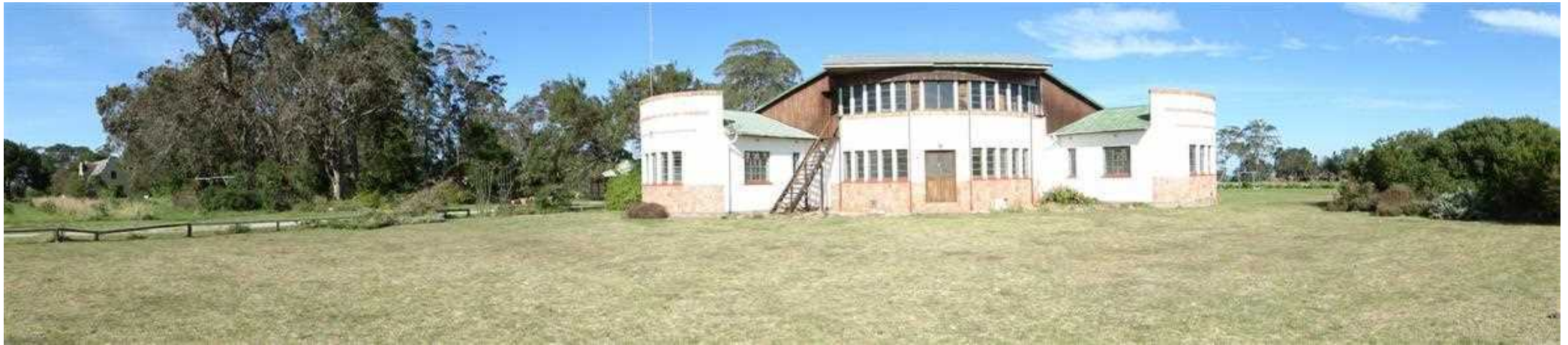
Photo 7: Main, north-facing façade of the historic farmstead (proposed guesthouse) with later added first storey to be removed.
