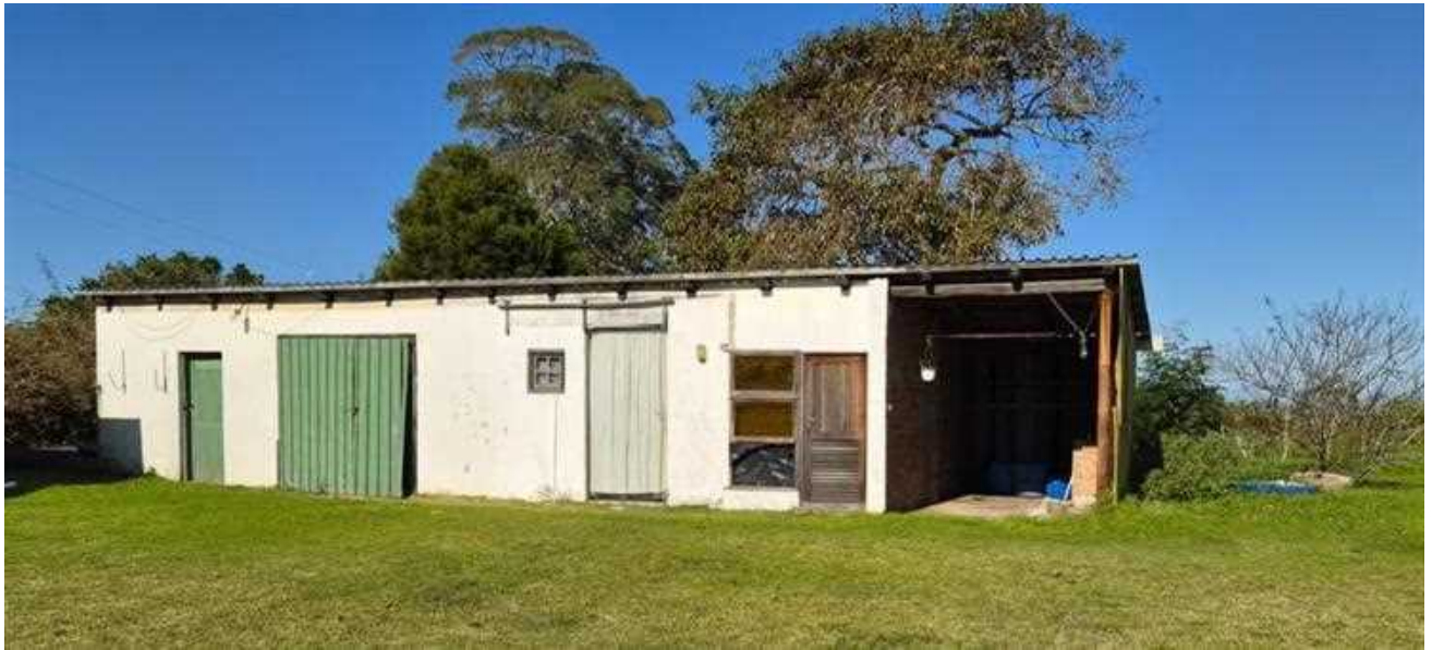
Photo 2: Building B, existing outbuildings located to the rear of the historic farmhouse, which is proposed to become a kitchen and laundry room.
