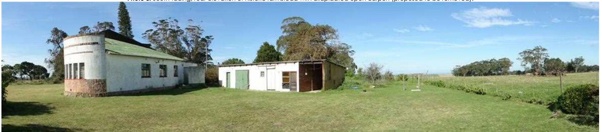
Photo 9: Side (west-facing) elevation of historic farmstead with dilapidated outbuilding (to be repurposed) to rear.
