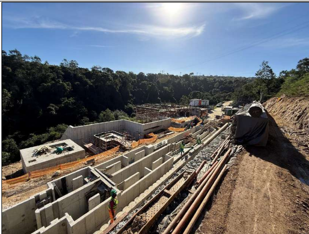
FIGURE 11: UPGRADING OF THE THEMBALETHU NO. 6 SEWER PUMP STATION
