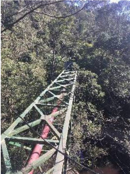
Figure 3-20: Existing pipe bridge
