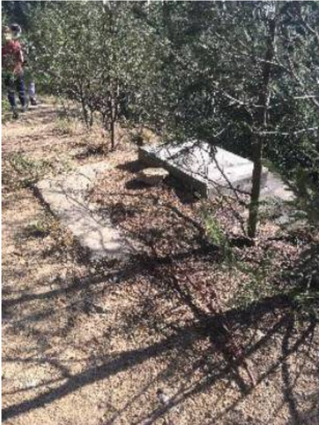
Figure 3-24: Existing infrastructure on pipe route
