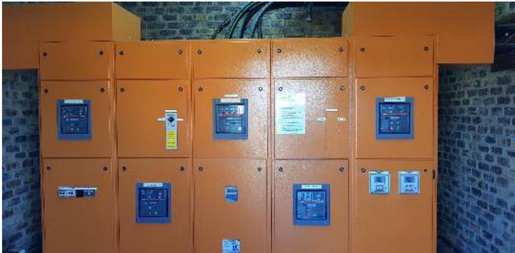
Figure 4-12: Proposed Main LV Incoming Section
