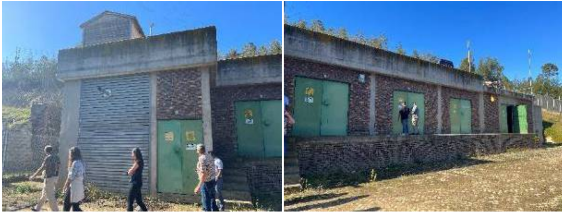
Figure 3-8: Existing pump station electrical rooms
