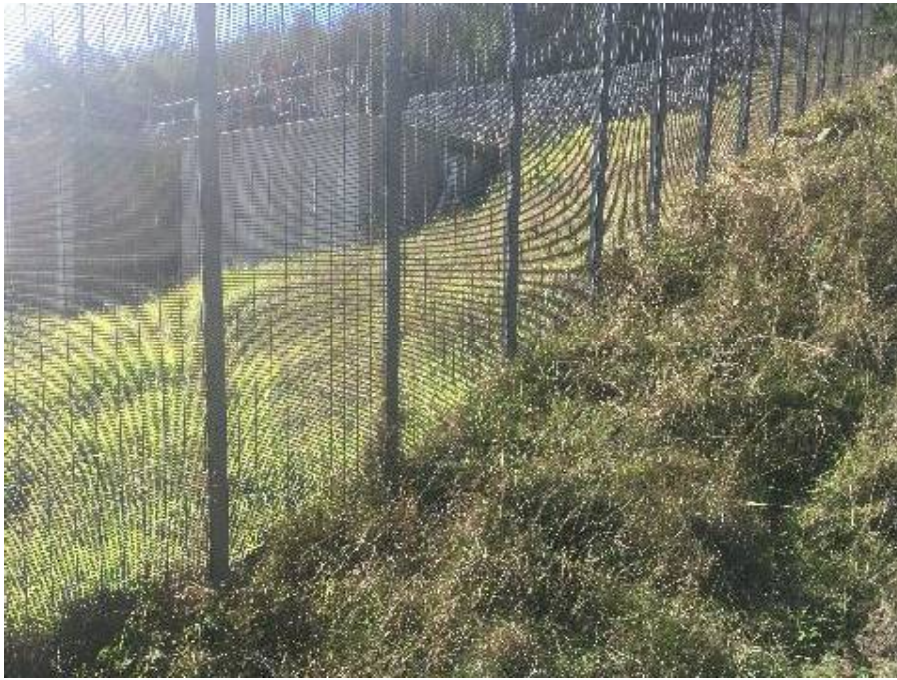
Figure 3-4: Photo of existing ground slope and gabions
