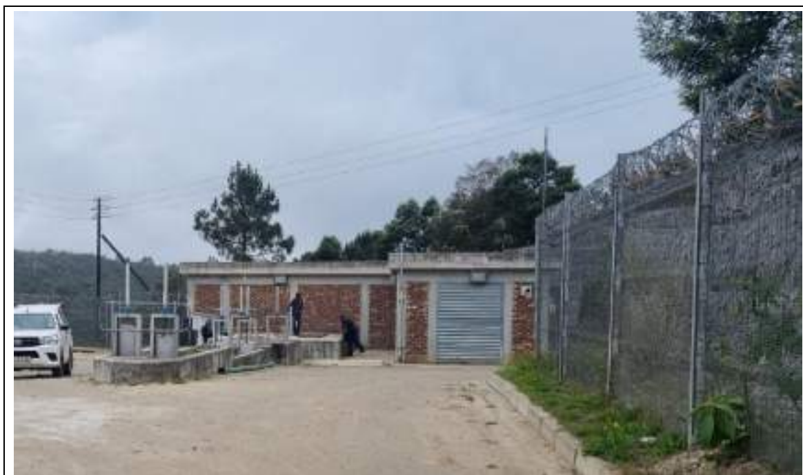
Figure 4 : General Site Picture of the Existing Thembaletu PS 7 Inlet Works
