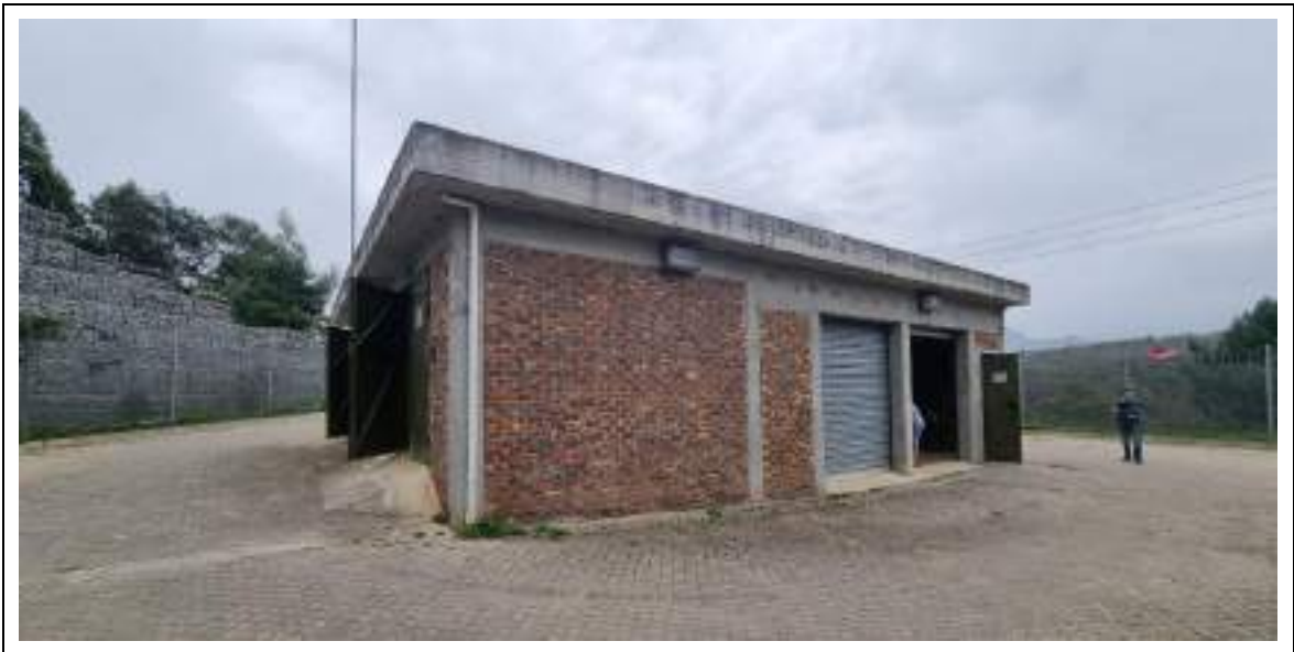
Figure 7 : Picture of the Pump Station Pump House
