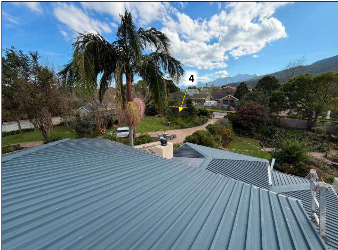
Figure 25: View northwest to west
