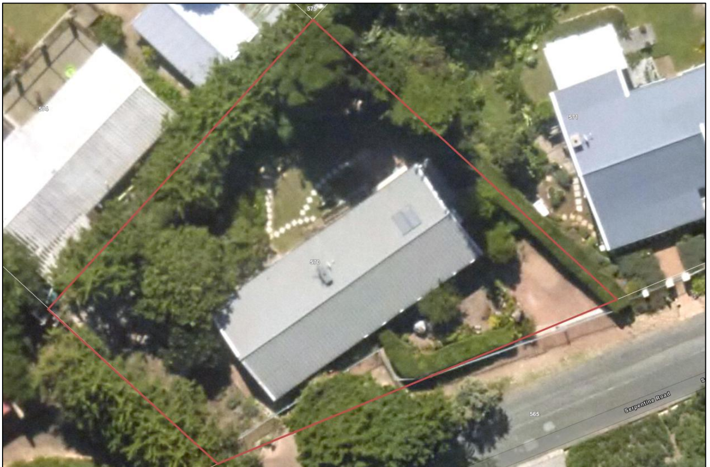
Figure 2: Enlarged aerial photograph
