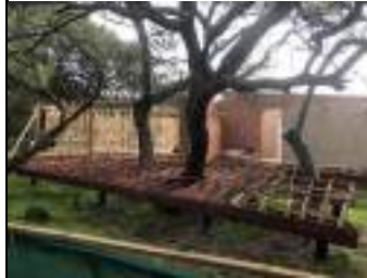
Figure 14 Tree roots were protected by pad foundations.
