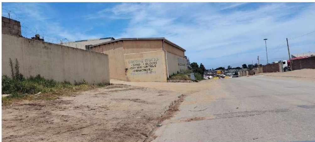
Photo 2 The photo shows the building on Erf 16815 (George Bricks) that encroaches unto the street reserve of Binne Street.
