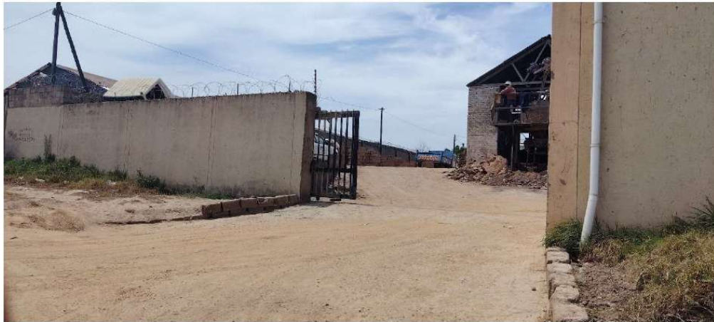
Photo 1 Erf 16815 is used for making cement bricks. The encroaching building is on the right side of the photo.
