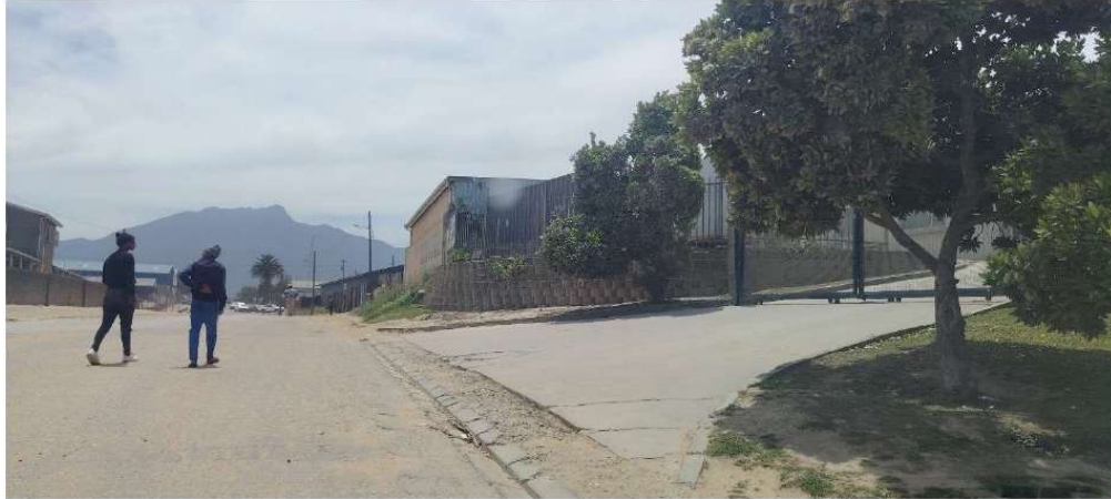
Photo 5 - showing the encroachment of the building on Erf 16815 unto the street reserve.
