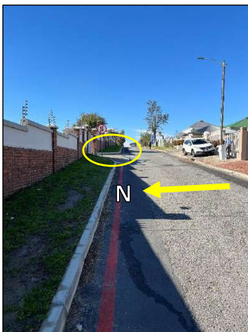
Figure 15: Street facade to the north
