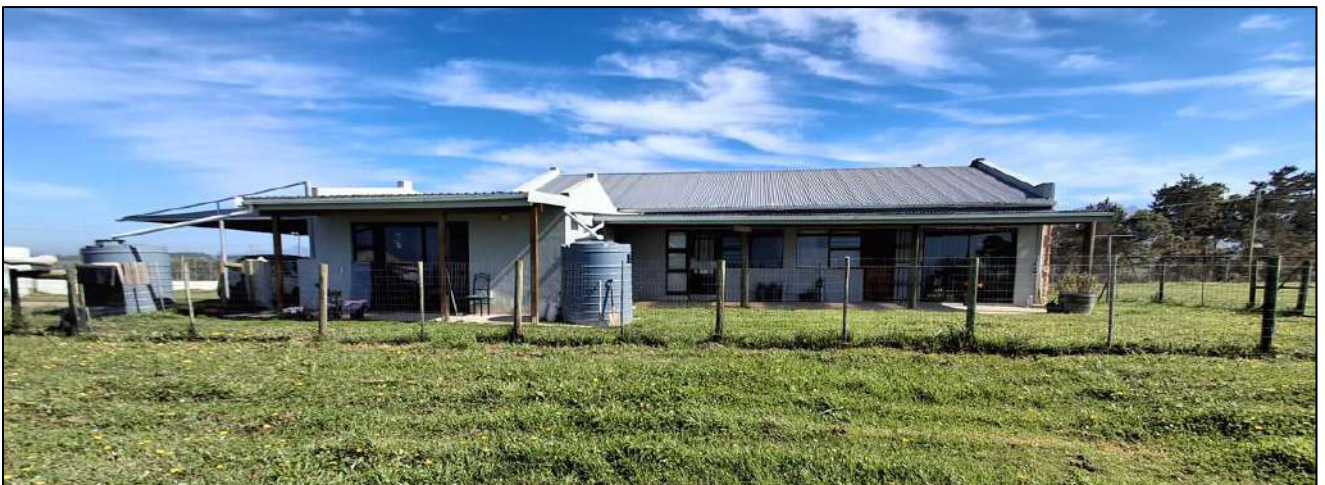
View of the second dwelling unit from the south – see two covered stoeps with a floor area of 36m 2 .
