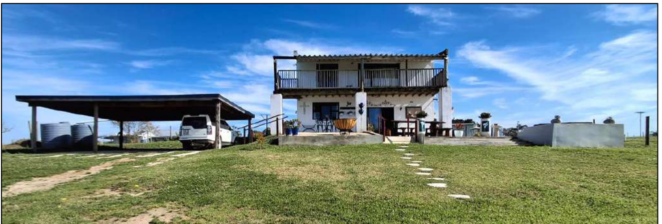
Primary dwelling house as seen from the south.
