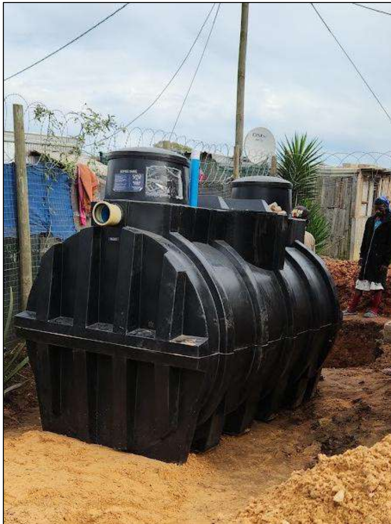
FIGURE 6: 3700 LITRE BUFFALO TANK. DURING INSTALLATION
